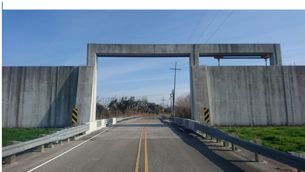
Louisiana flood defence wall
