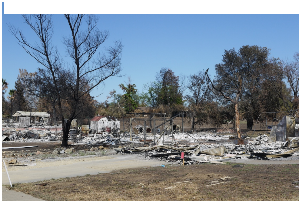
Remains of housing estate after Carr fire in Redding, California
