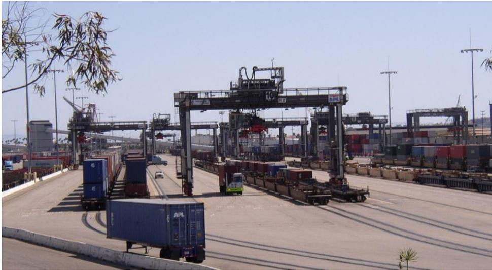
**Figure 3: Intermodal ship-to-rail transfer of containerised cargos, port in Long Beach, California<sup>10</sup>**
