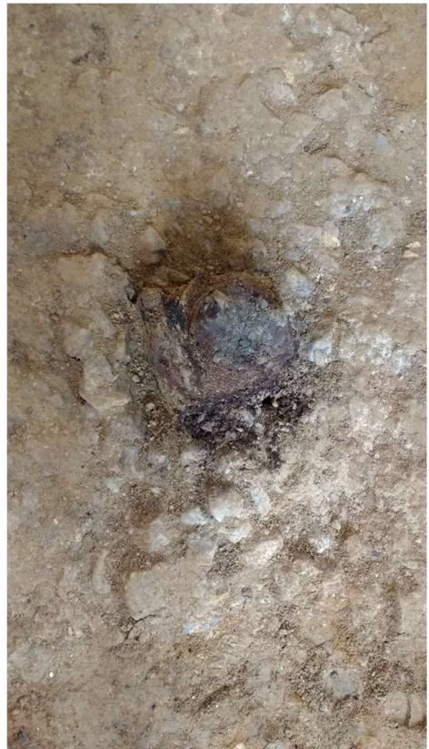
Figure 6: Chapel floor with existing timber posts
