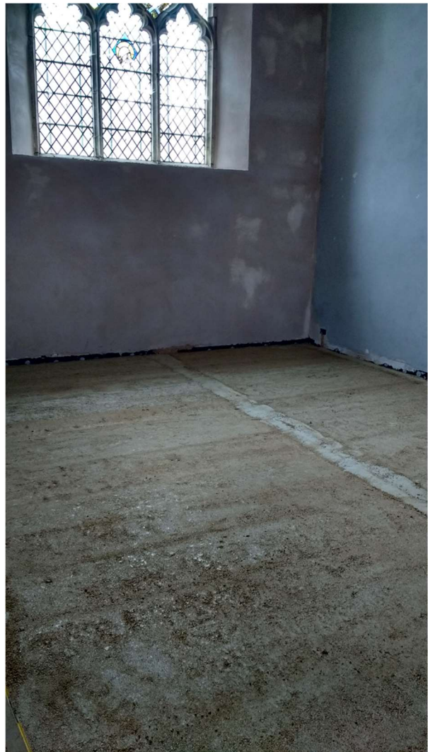
Figure 8: Chapel floor lime screed
