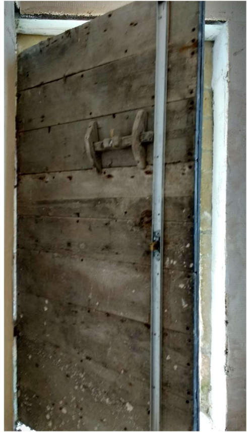
Figure 3: Chapel door internally
