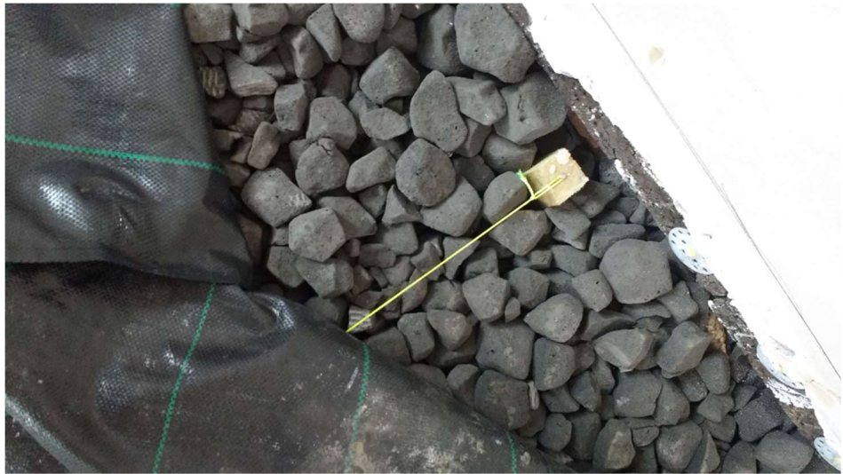
Figure 7: Chapel floor insulating hardcore
