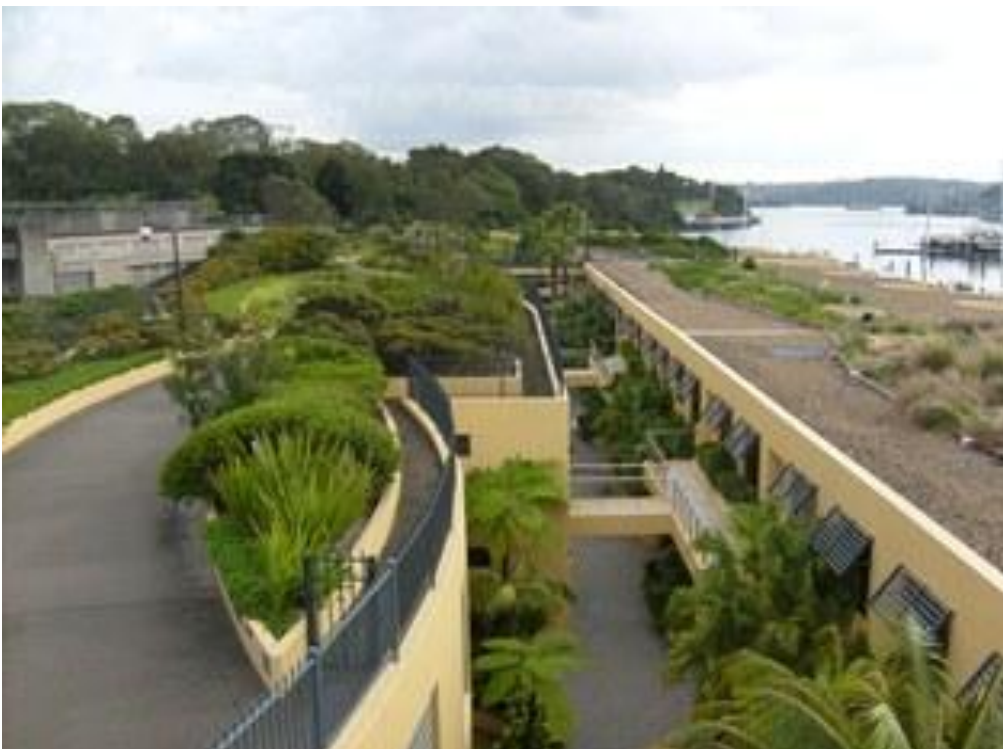
Plate 2 Wharf Terrace Woolloomooloo Sydney - intensive green roof
