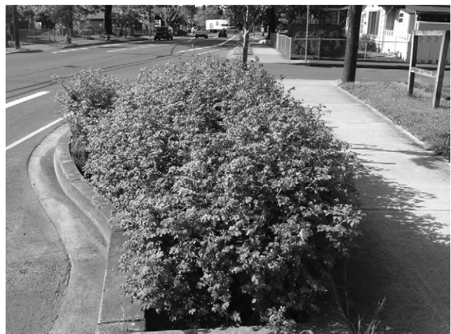
Figure 6. Bioswale with kerb-cut in the USA
