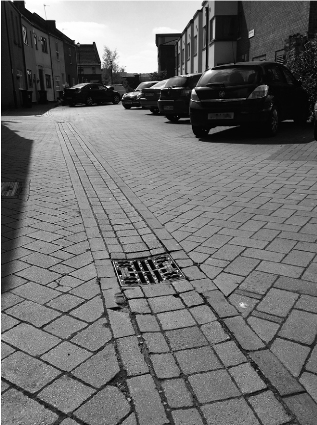
Figure 2. Permeable paving in the UK
