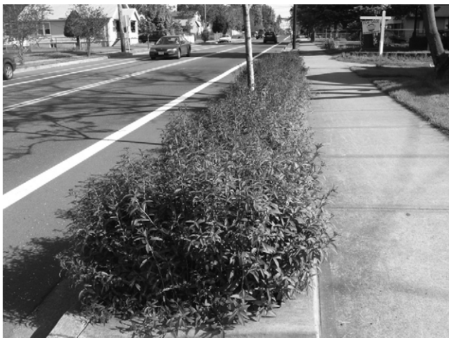
Figure 7. Bioswale without kerb-cut in the USA
