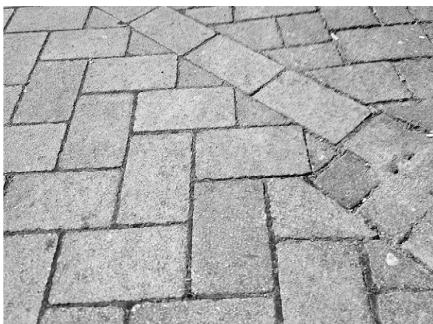
Figure 5. Permeable paving in the UK – close-up
