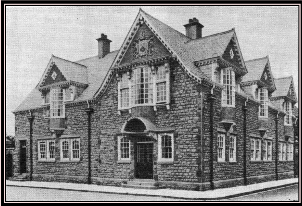
FBB's Westward House, Shirehampton (1906), demolished in 1952
