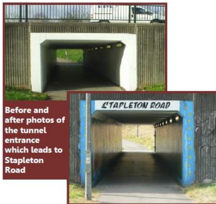
Figure 1 - Photograph from monitoring agreement showing one of the underpass tunnels before and after the completion of the scheme
