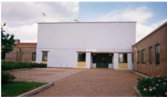
Buildings (e.g. hospital, shed, brick wall)
