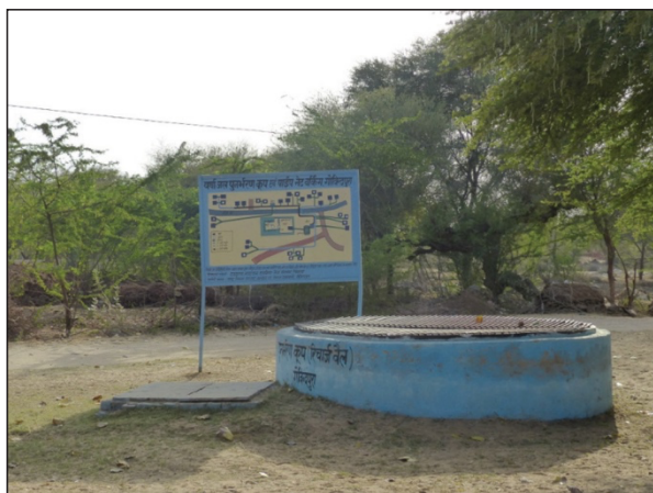
Figure 6. Recharge Well and Installation
