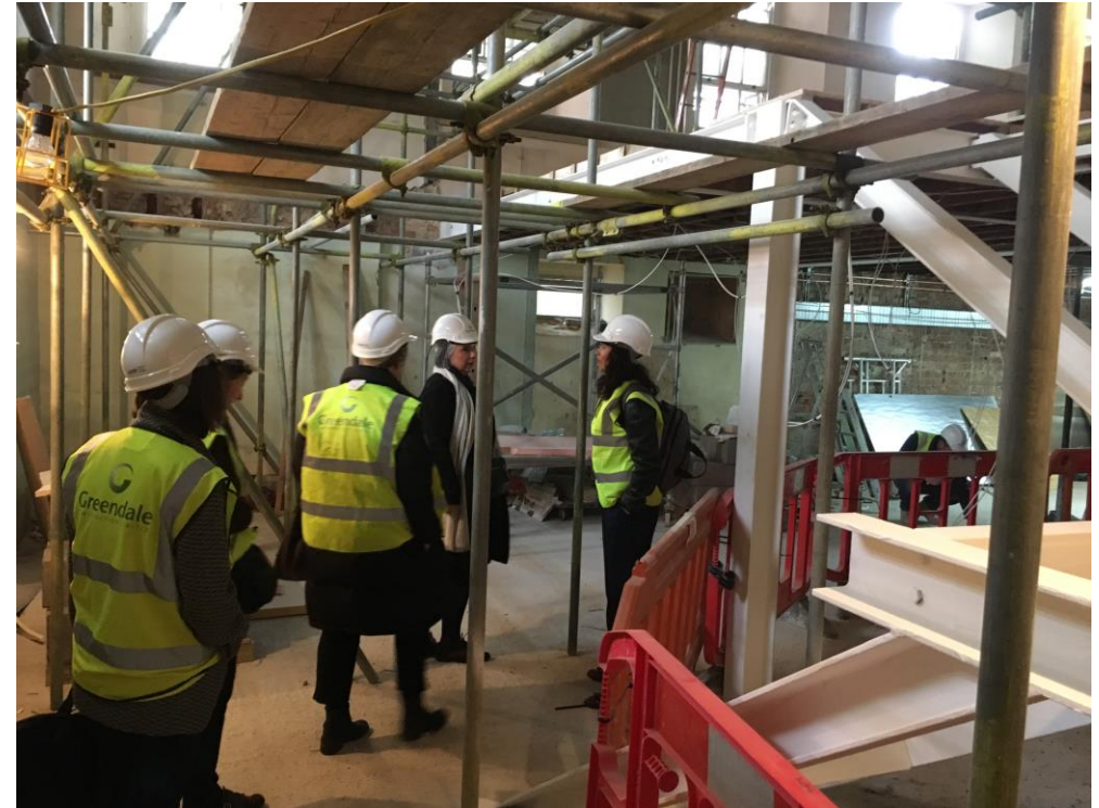
The project team on site during construction
