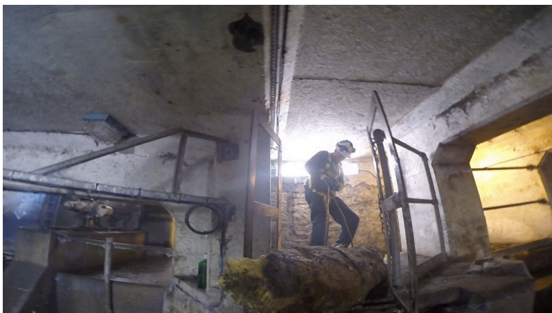
Figure 2. Repetitive, mundane, yet vital maintenance: pulling a log out of the River Frome (underneath Bristol City Centre).
