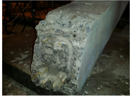
Figure 6.11 Picture showing the shear failure of Beam 7
