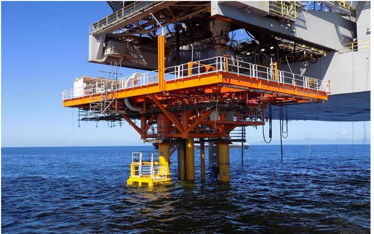
**Figure 3.2:** Conductor supported production platform (Source: Gill, 2019)
