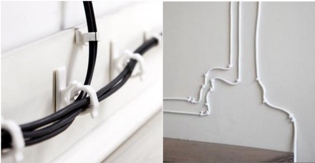
Figure 21 Wires clipped to wall
