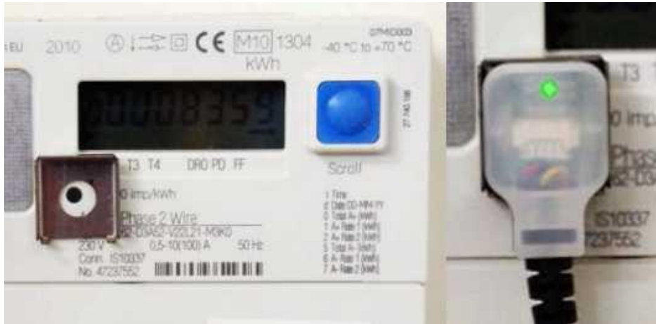
Figure 6 Pulse counter mounting on a meter
