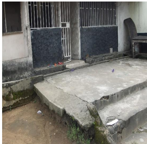
f) Self constructed drainage close to home entrance
