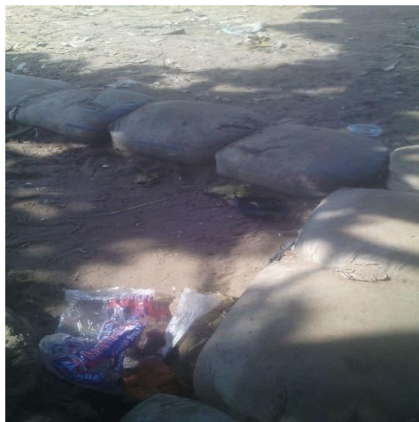
b) Sandbags arranged few meters from building to prevent flood waters
