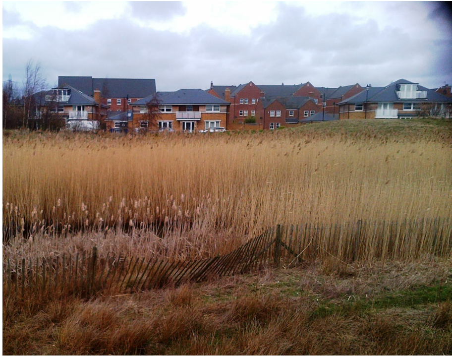
Fig. 1. Case study site 1, England: A SuDS retention pond close to a new housing development, planted with reeds to aid with the uptake and filtration of stormwater, foster biodiversity and provide amenity opportunities. (Credit: Jessica Lamond, 2017).
