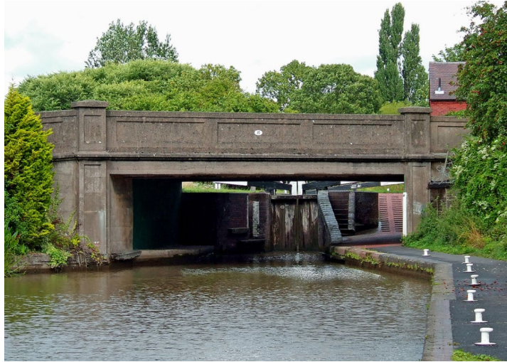
The current Bilford Bridge 5
