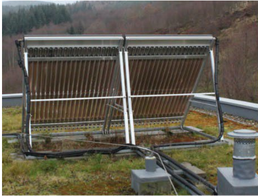
Solar thermal hot water system and control
