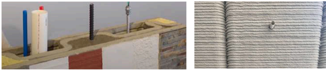
Fig 11. Cavities layout to incorporate services.
