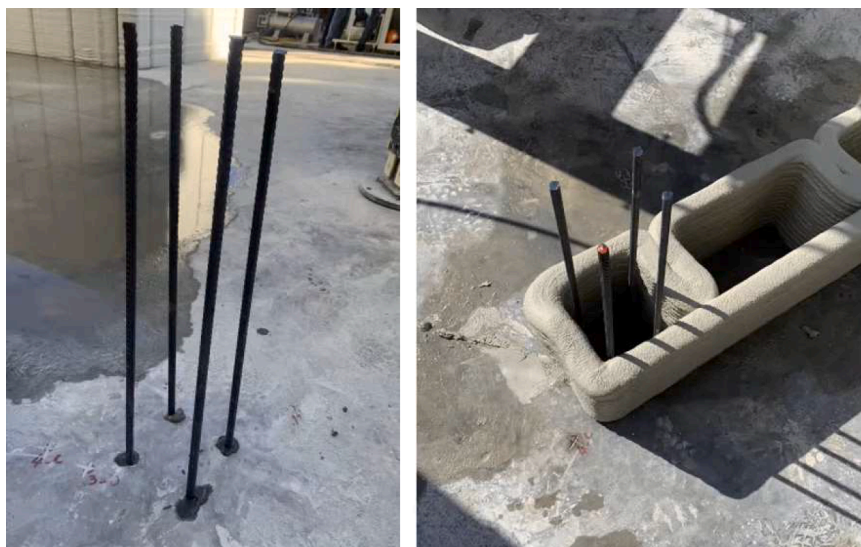
Fig. 10. Integrating steel reinforcement to 3DPC house.
