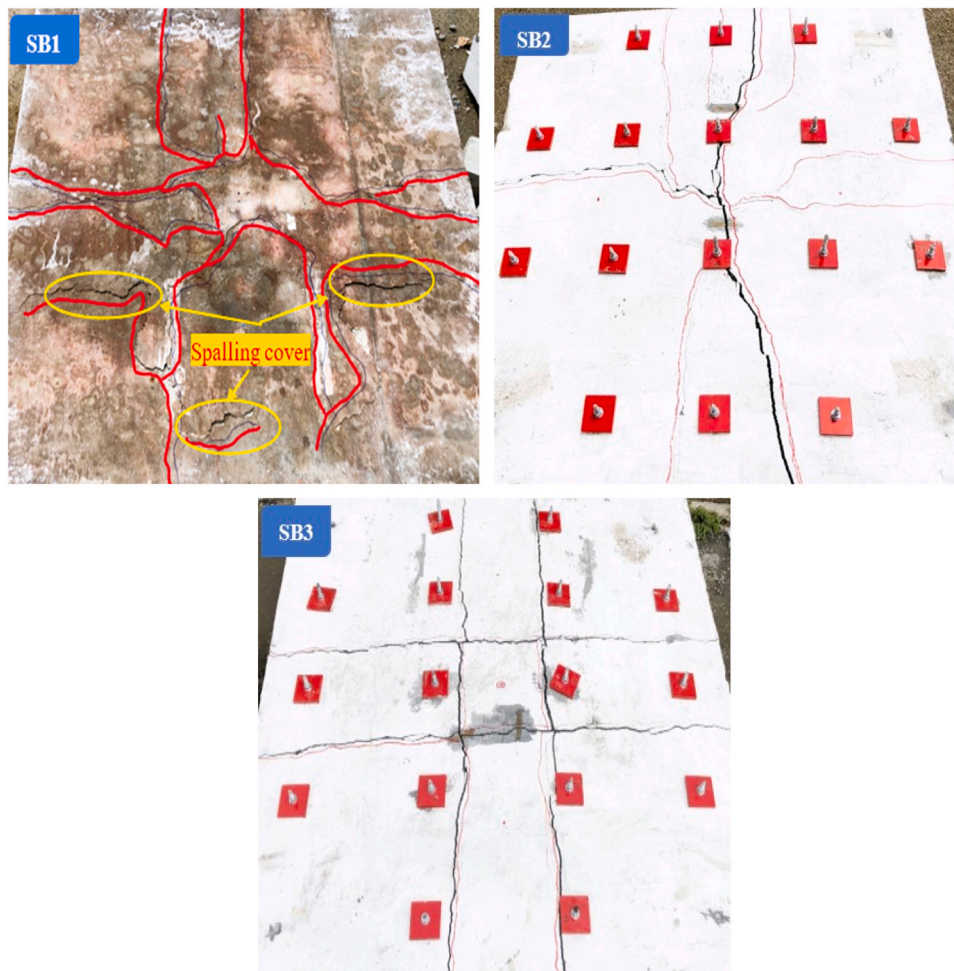
Fig. 12. Crack patterns on the bottom face (tension side) of specimens.
