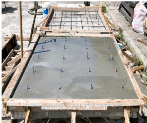
Casting the UHPFRC
