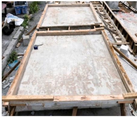
Fabricating the mould
