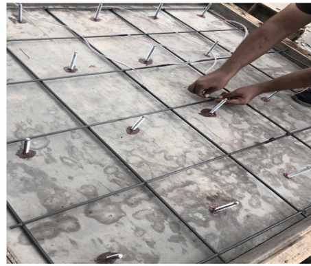
Reinforcing the jacket with CFRP rods
