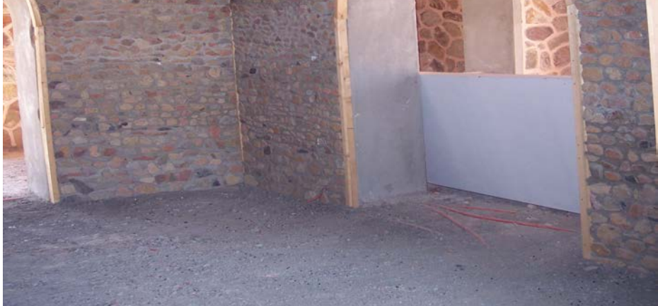
Foundations of rocks and earth mortar
