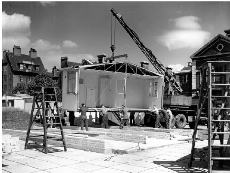
Figure 3. Prefabricated volumetric module at London Exhibition, 1945 [16].
