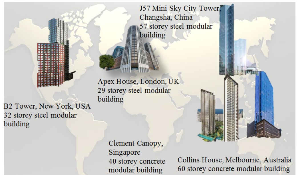
Figure 7. High-rise modular buildings [46].
