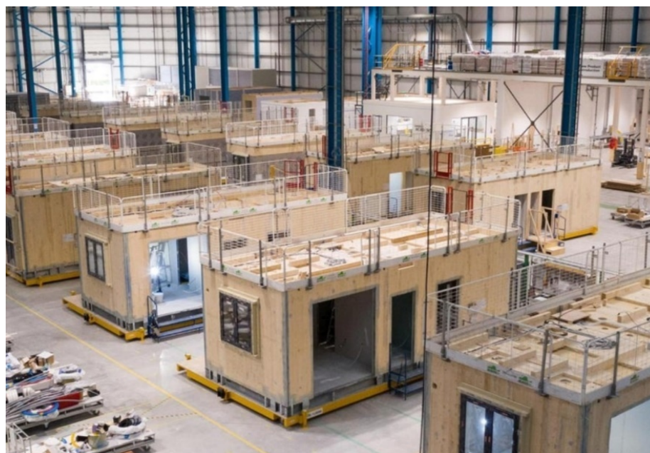
Figure 1. Prefabricated modules in a factory [14].
