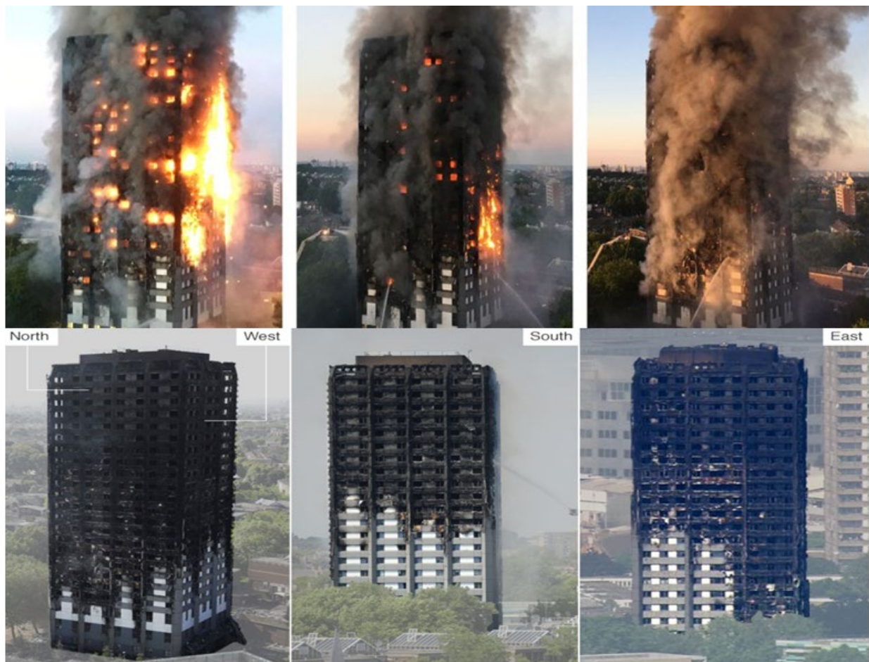
Figure 9. Fire accident in Grenfell Tower, UK [58].
