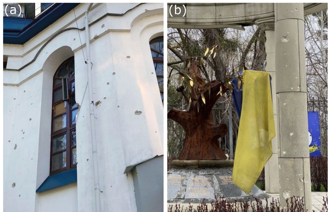
Fig 1. (a) Shrapnel damage to the facade of the St Nicholas Church caused by Russian shelling in the town of Irpin, a suburb to the NW of Kyiv in Northern Ukraine [2]. (b) Impact damage to columns of the Alley of ATO Heroes memorial, also in Irpin. It is reported to have been caused by small arms fire from Russian forces in February 2022 [1, 2].
