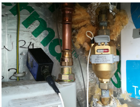
Figure 4. Silhouette logger (black box) attached to water meter. Used with permission of the creator.
