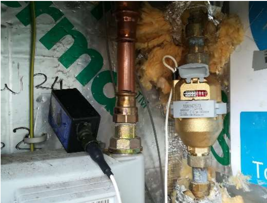
Figure 3-7 Siloette logger (black box) attached to AMR meter via white splitter cable (Source: author)
