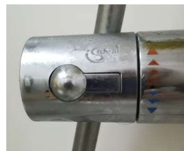
Figure 3-7 Shower thermostatic control (Source: author)
