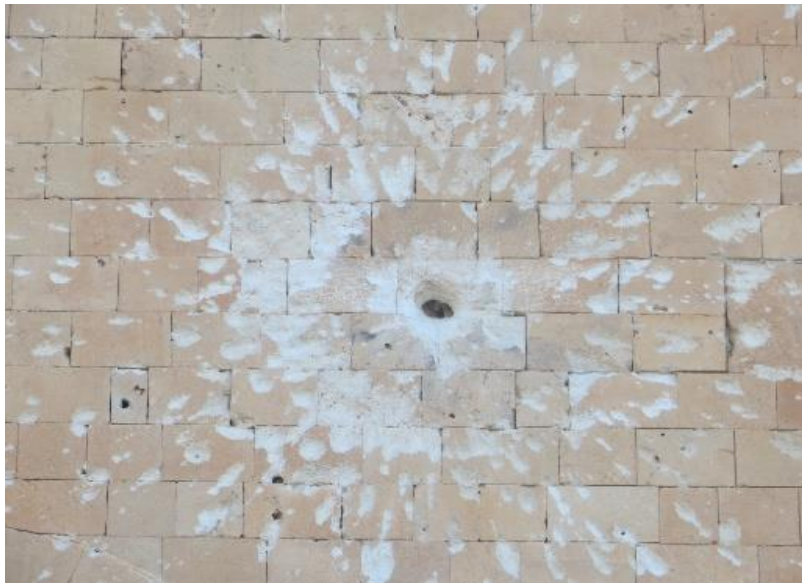
Figure 7.18: Radial scarring around the RPG Hit perpendicular to the central hole indicating the direction of travel of the RPG.
