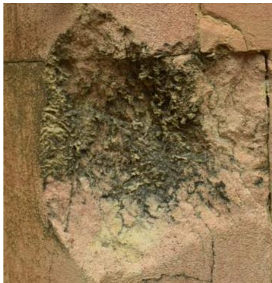
Figure 3.30: Image of the black weathering formation in an impact crater on column 8 side 2, north facing.
