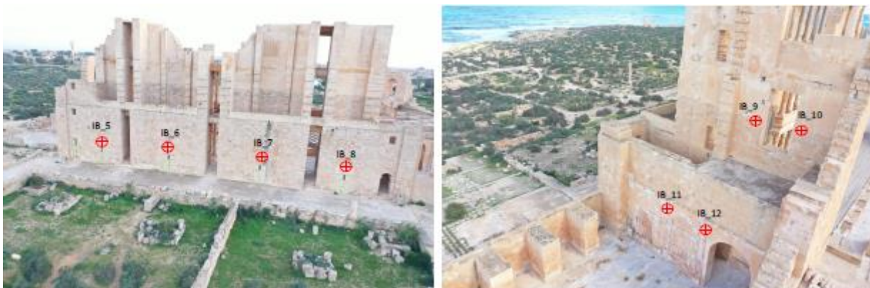
Figure 7.21: Locations of temperature sensors (North Wall) IB 5 and IB 10 (West wall).
