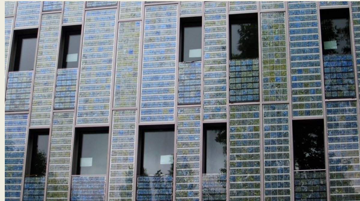
La Citta Vita (2011) Solar facade [photograph]. At: Flickr [online]. Available from: go.uwe.ac.uk/SolarFacade [Accessed 17 June 2023]. Licence: go.uwe.ac.uk/CCBYSA2
