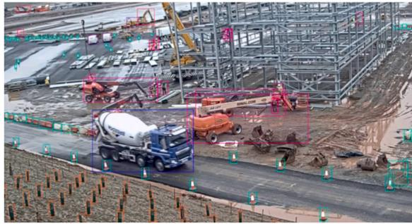
Fig. 6. Identification of construction objects on construction site (CVAT).
