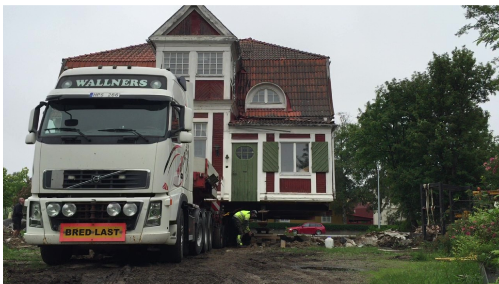
Figure 2. Historic house being lifted, to move from its site at Teg in the city of Umeå Film Still Tonia Carless 2021
