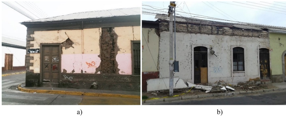
Fig. 7 a Poor interlocking connection of the adobe bricks at intersections; b impulsive nature of the roofing structure
