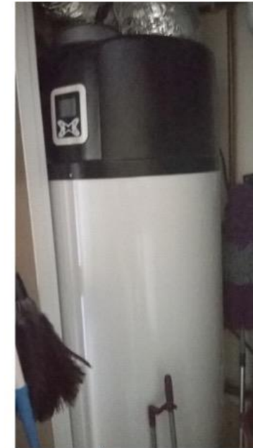
Thermal water tank And control
