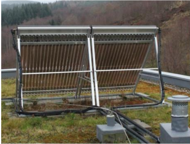
Solar thermal hot water system and control
