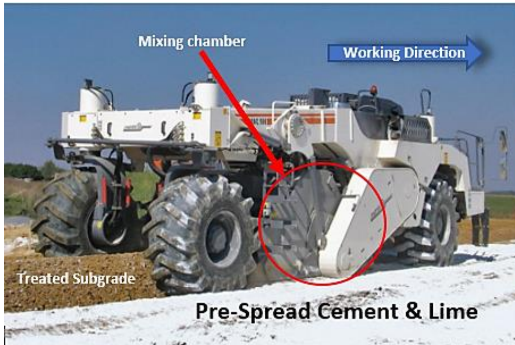
Insitu soil stabilisation process (Wirtgen-group.com, 2021)
