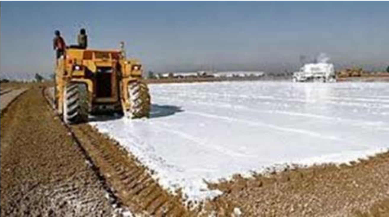
Figure 2.11: Lime stabilisation process in road construction (Saranya et al. , 2017)
