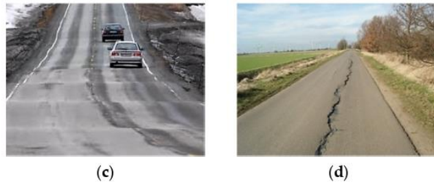
Figure 2. (a) Typical wet expansive soil [14]; (b) typical dry expansive soil [15]; (c) uplifting of flexible pavement due to expansive soil [16]; (d) typical longitudinal crack developed on pavements over expansive clays [17].
