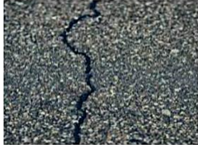
Transverse Cracking
