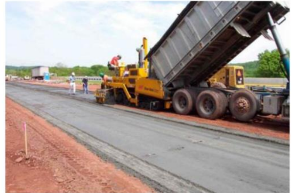
Fig. 15. Fly ash stabilisation process in road construction (Beeghly et al., 2003).
