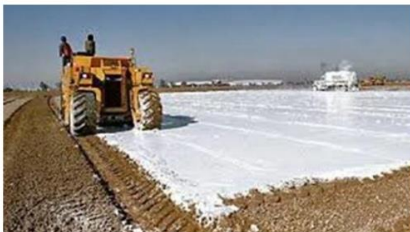
Fig. 14. Lime stabilisation process in road construction (Saranya et al., 2017).
