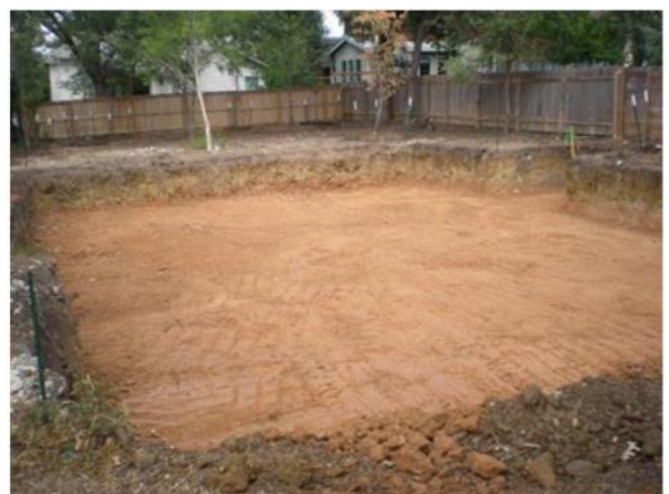
Fig. 11. Soil removed and ready for backfill (Capital geotechnical services PLLC).
