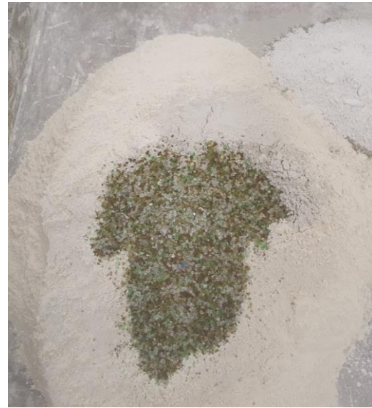
Recycled glass grits and other binders added to subgrade material during the mixing process
