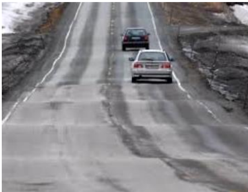
Figure 1.5:Uplifting of flexible pavement (White et al. , 2021)
