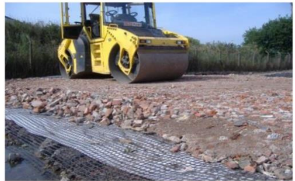
Fig. 16. Construction and demolition waste, Geogrid and textile used in road construction (ABG Geosynthetics).
