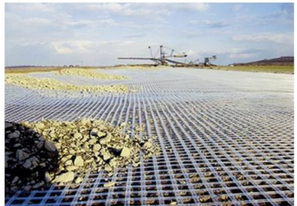
Fig. 9. Soil reinforced with Geogrids(Kiganda, 2016).
