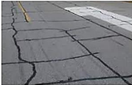
Block Cracking
