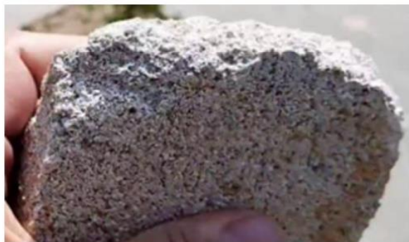
Fig. 19. Soil stabilised with polymer for road construction (K31 Roads, 2018).
