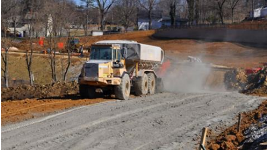
Figure 2.9: Cement stabilisation process in road construction (Pleasants Construction, Inc, 2020)
