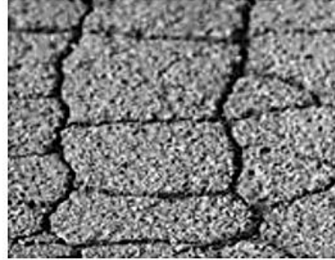
Alligator Cracking
