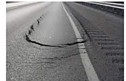
Slippage Cracking
