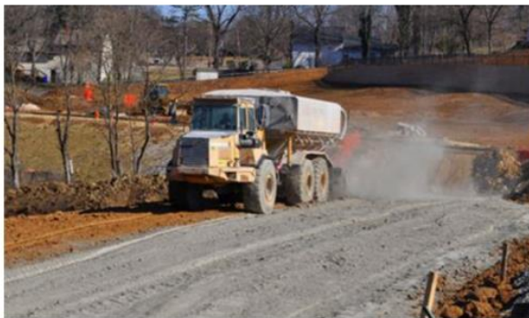
Fig. 13. Cement stabilisation process in road construction (Pleasants Construction, Inc).
