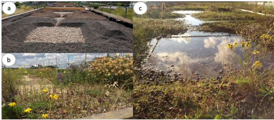
Fig. 2. The brownfield mosaic ecomimicry extensive green roof included locally typical substrates to create heterogeneous thermal, moisture and organic conditions and encourage habitat mosaic development (a). These were applied in varied depths to create microtopography and structural diversity, to increase niches for plants and provide refugia for biota during hot, dry or cold spells. Locally-attuned, diverse wildflower assemblages were planted (b) to provide a broad range of foraging resources, and enhance habitat heterogeneity through structurally complex plant architecture. In addition, innovative drainage mechanisms were used to recreate seasonally wet brownfield habitat niches (c).
