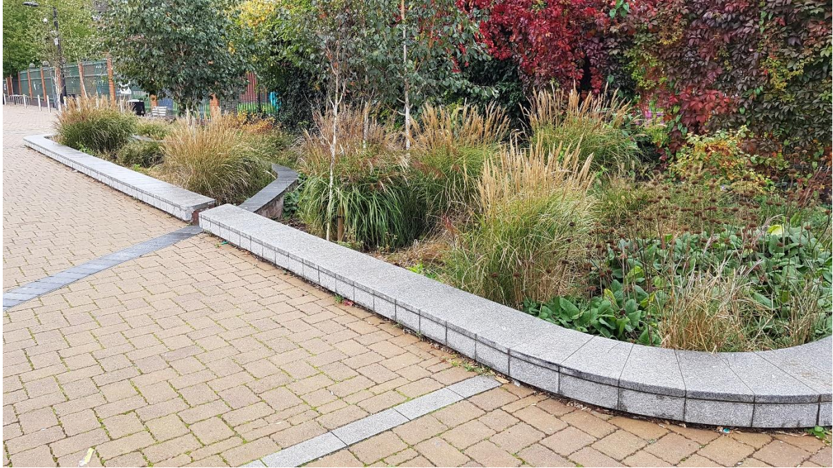
Figure 5. An example of a well-adopted Sustainable Drainage System (SuDS). Consideration for the SuDS legacy means that it is well-managed and considered to be a valuable asset by the local community.
