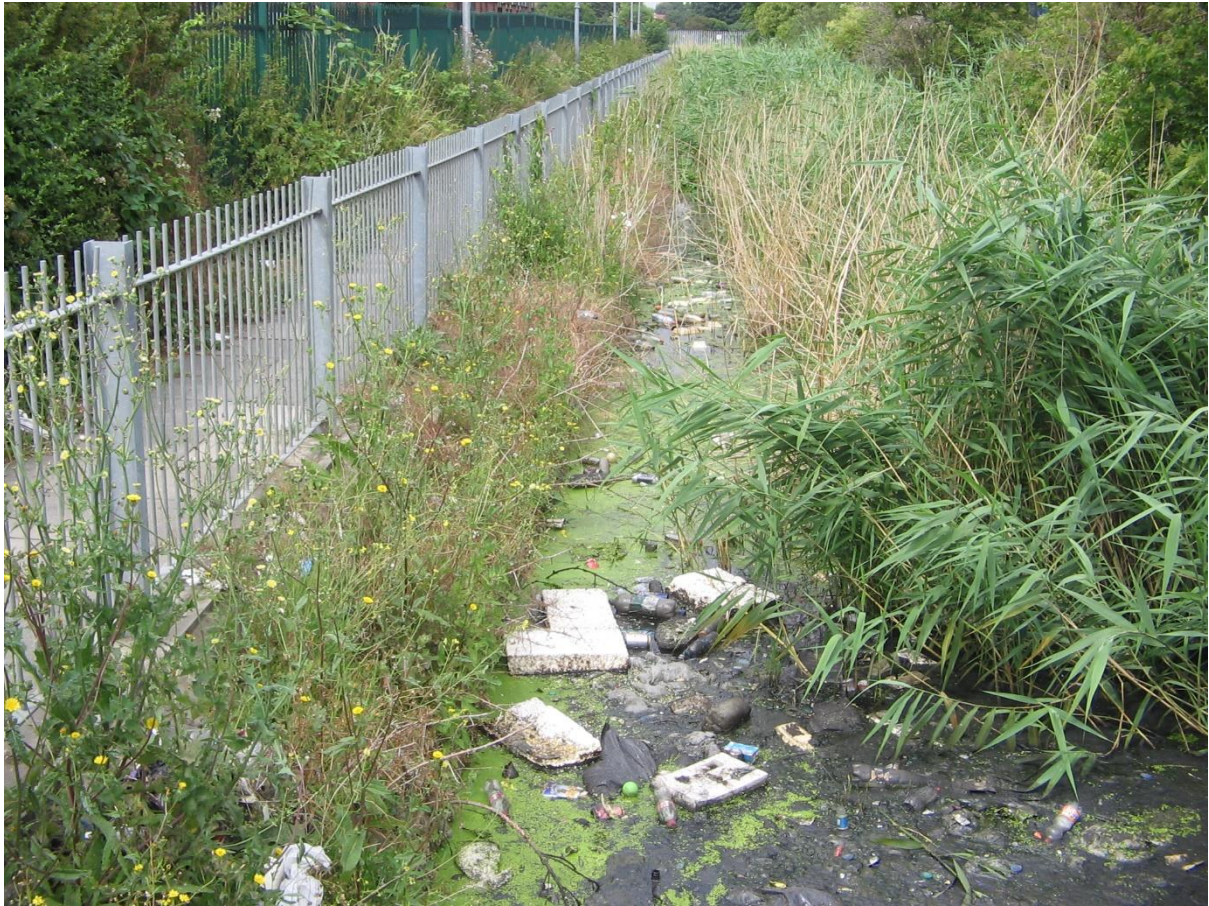
Figure 2. Example of a nature-based solution with inadequate legacy management. The legacy of this stormwater management ditch was not considered in relation to appropriate management. As such, it is seen as a negative feature of the area and is used for dumping of trash. © Stuart Connop
