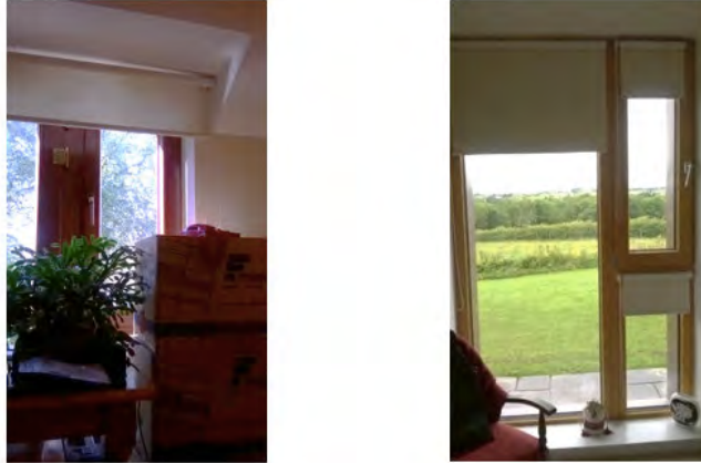
Figure 2. Comparison of blind arrangement in SL project (left) and HA project (right)
