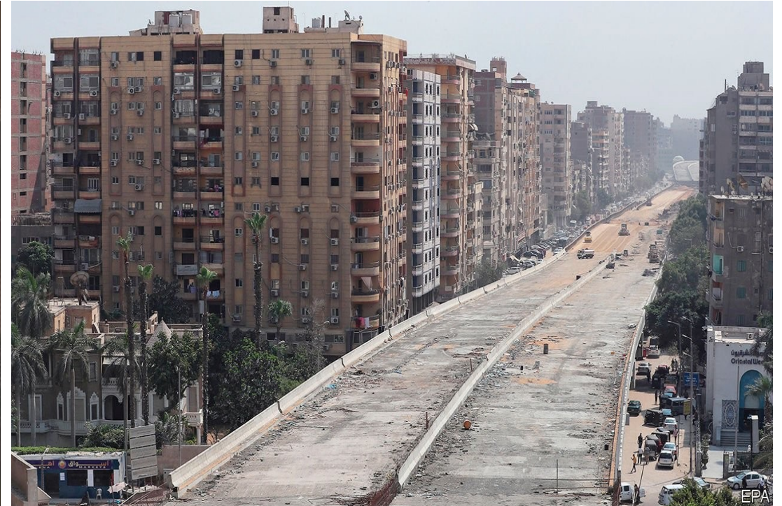
Proposed Bridge (currently under construction)
