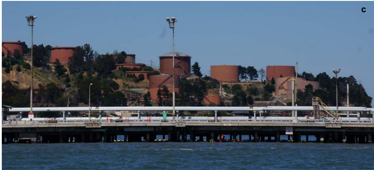
Figure 8. San Francisco Bay Area TFS hub terminal examples. a) Nustar rail/pipeline/marine terminal. b) Shell marine/pipeline terminal. c) Chevron marine/pipeline terminal.
