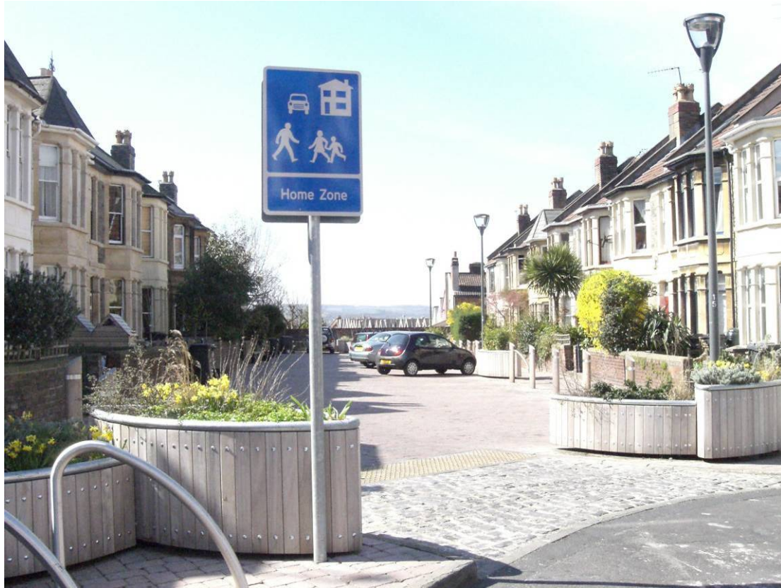
Plate 1.1: Stackpool Rd Cul-de-Sac HZ as Constructed
