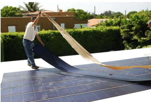
Fig. 2 Thin film photovoltaic modules. Note. From Thin Film Flexible Solar PV Installation 2 [Photograph], by Ken Fields, 2008, Flickr, ( https://www.flickr.com/photos/51925339@N05/4783039248 ). CC BY-SA 2.0.
