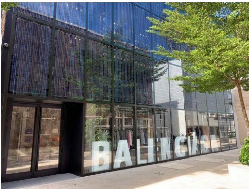
Fig. 1 Photovoltaic glass façade integrating crystalline silicon solar cells. Note. From Balenciaga Miami Design District [Photograph], by Phillip Pessar, 2018, Flickr, ( https://www.flickr.com/photos/25955895@N03/46276576481 ). CC BY 2.0.
