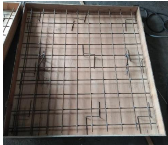
(b) lower slab reinforcement
