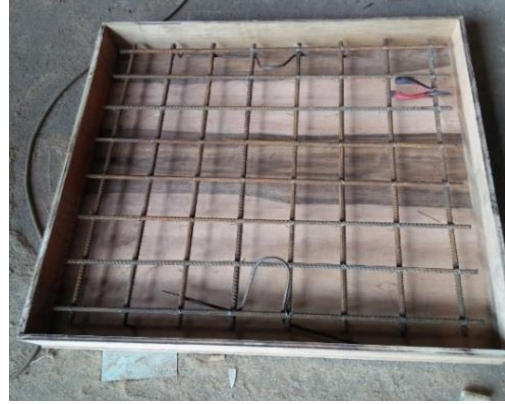
(a) upper slab reinforcement
