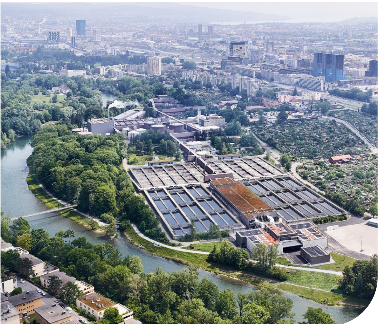
Figure 18: The Werdhölzli sewage treatment plant in Zurich. Analysis of wastewater can indicate levels of COVID-19 in the population. (Photo: City of Zurich)
